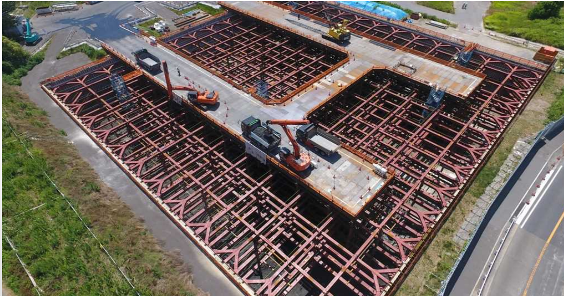
※Under construction(Project period : FY2017- FY2021(planned))
